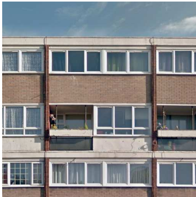
Figure 1. Ornamental brick pilasters in the façade of four-storey block of maisonettes, LCC Lockesley Estate, 1954. Google Street View, 2020.
