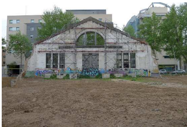
Figure 2. On-site works for a public facility by recovering an old factory facade as a trace from the industrial heritage. Image: Marta Serra-Permanyer, 2021.
