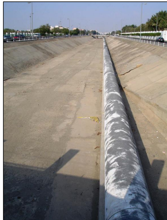
Figure 9. A Channel Collecting Stormwater (Jeddah Strategic Plan, 2009)
