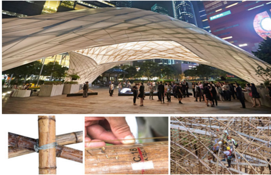
Figure 11. The construction process of ZCB Bamboo Pavilion CUHK (Crolla, 2017)
