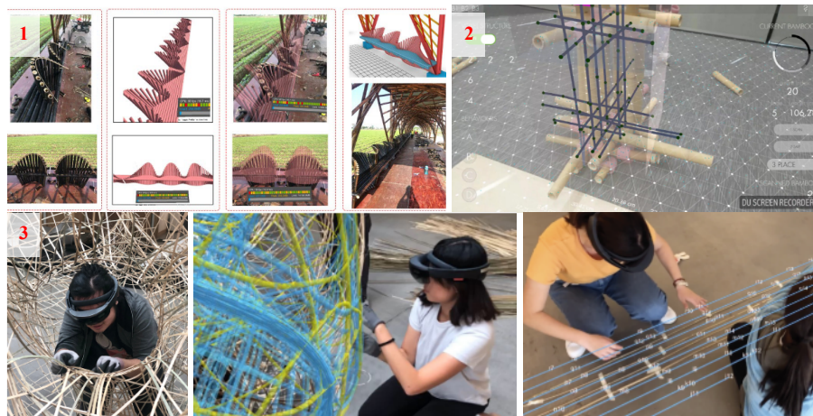
Figure 17. Mixed reality applications in the fabrication of bamboo structures: 1) Bamboo Pavilion Diecui Gallery in China (Kenan Sun, Tian Tian Lo, Xiangmin Guo, 2022), 2) Rawbot Bamboo project, a Mobile AR Assembly in UCL: United Kingdom (Wu et al. , 2019), 3) Argan Bamboo installation project in CUHK Hongkong (Goepel and Crolla, 2020)
